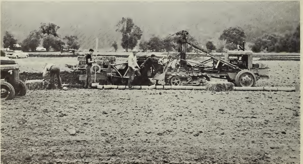
Photo 30.--Some fields are drained by a pattern-type tile system, Clatskanie Soil Conservation District, Oregon. SCS photo
